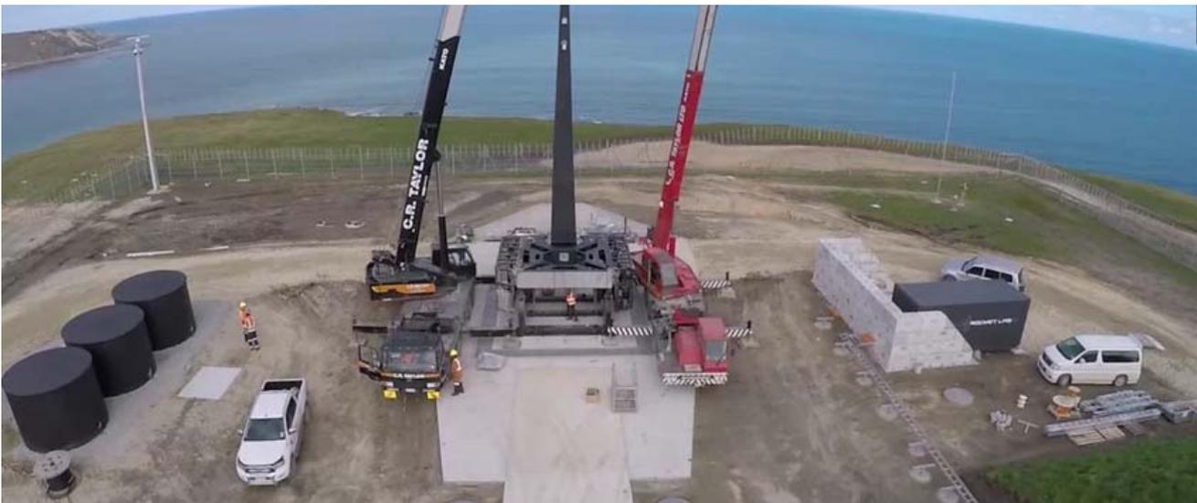
Facilities at Launch Complex 1 include a vehicle processing hangar where the vehicle will be prepared for launch as well as a 50 tonne launch platform. The platform will tilt forward to lift the rocket to a vertical position prior to launch.
